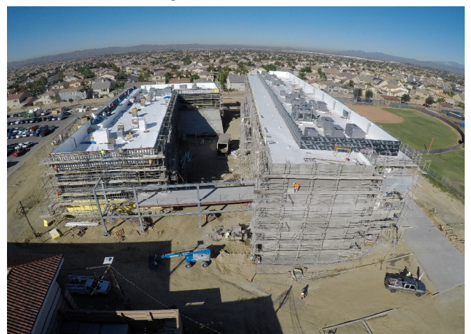
Buildings T1/T2 Exteriors
