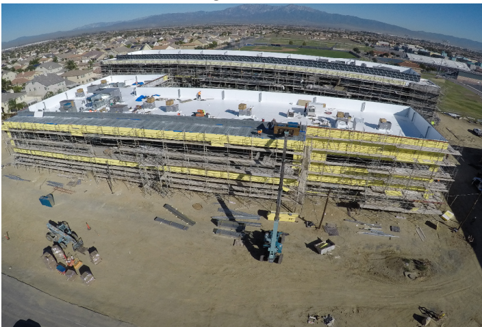
Building T2 Exterior
