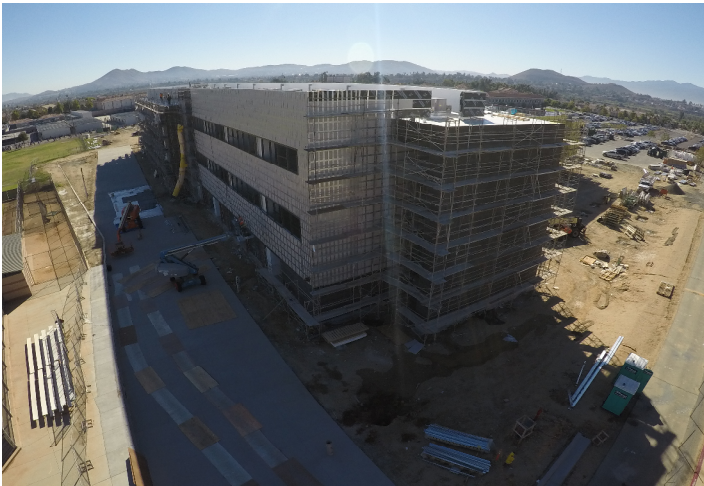
Building T1 Exterior
