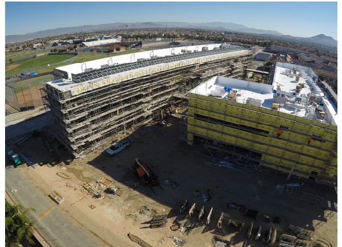
Buildings T1/T2 Exteriors
