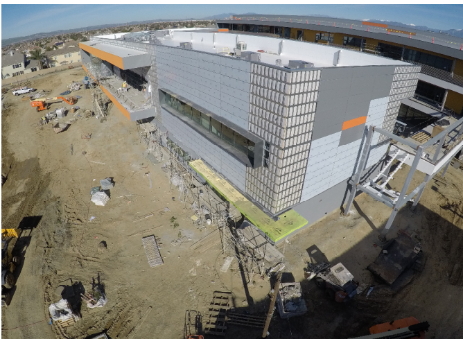
Building T2 Exterior
