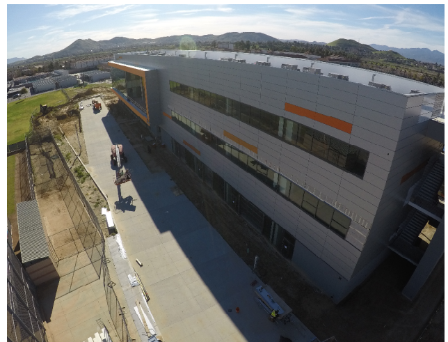
Buildings T1 Exterior
