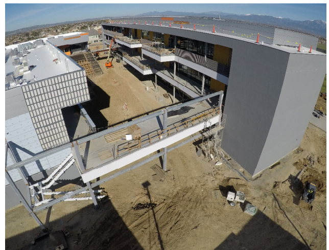
Building T1 Exterior
