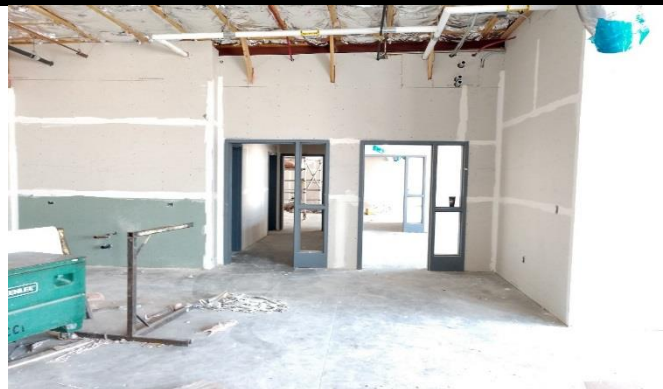
Drywall Building D
