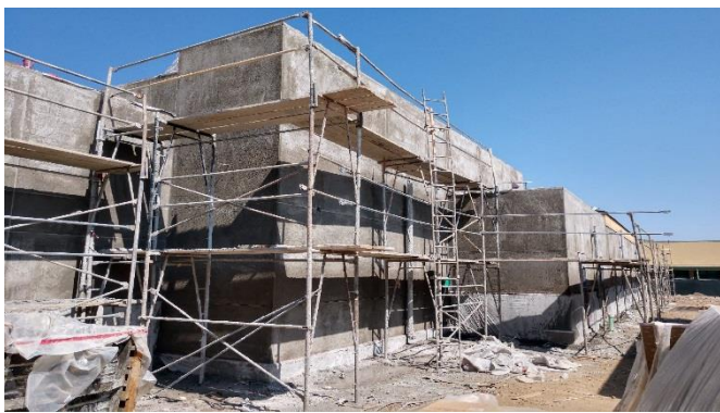
Building C, Brown Coat
