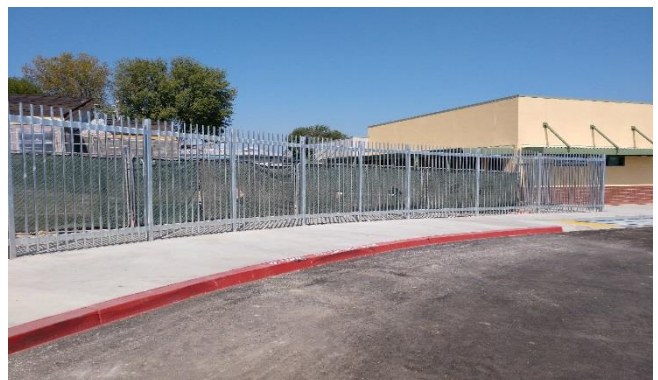
Parking lot Fencing
