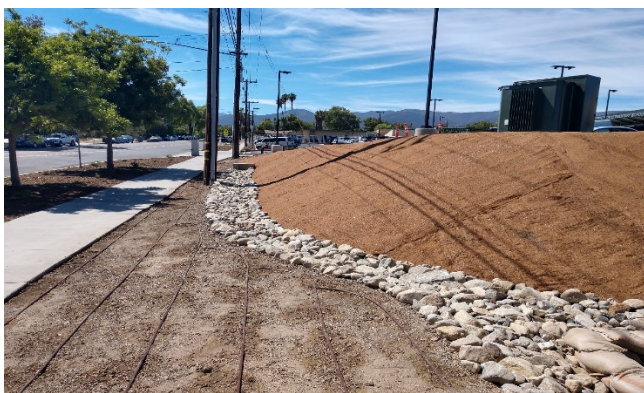
Landscaping in Progress
