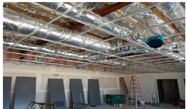
Building D T-Bar grid, doors painted
