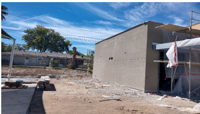
Building D color coat
