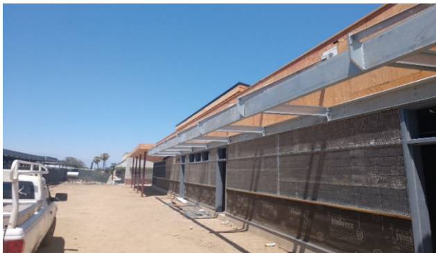
Canopy install and Lathing Building C
