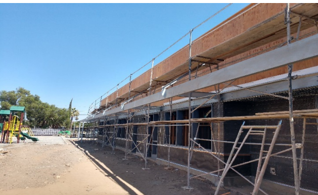
Windows/ Doors/ Lathing @ Building D
