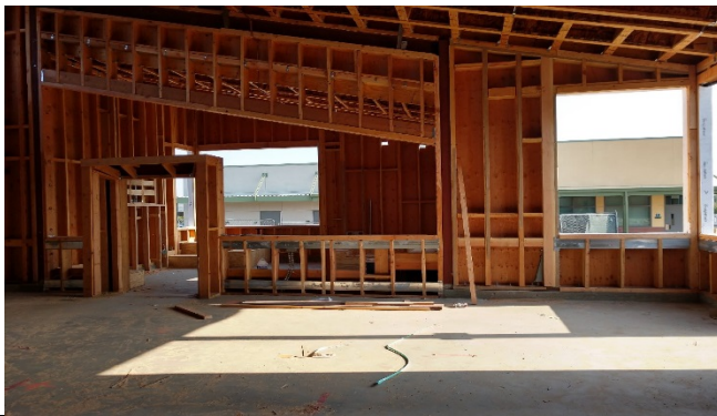
Framing at Building C Story room
