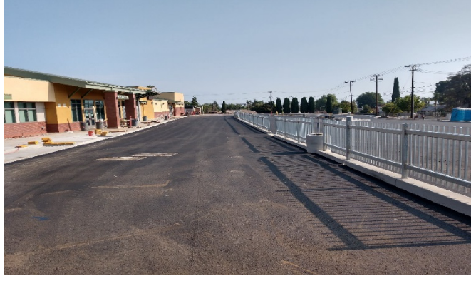
Asphalt @ Parking lot
