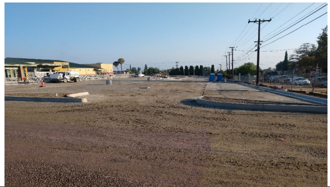
Base at Parking lot
