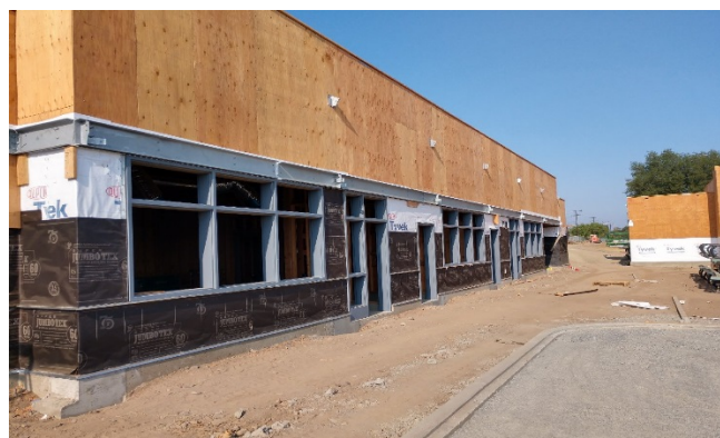
Windows / Doors/ Lathing @ Building D
