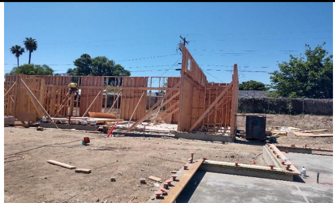
Building D - Wall Framing
