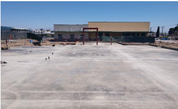
Slab Poured Building C
