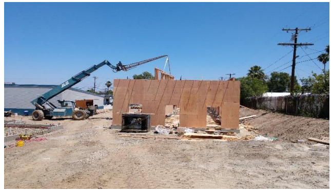
Standing walls - Building D
