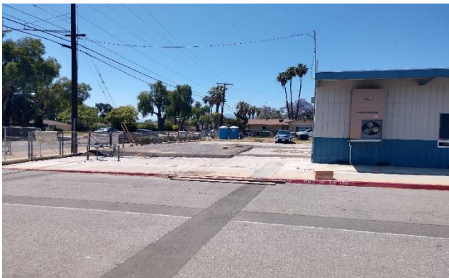
Site work - Moving out Portables
