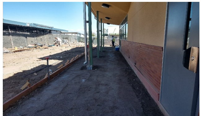
Building C sidewalk form work
