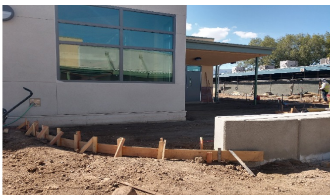
Building C sidewalk form work
