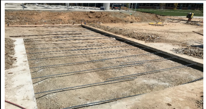
Rebar installation
