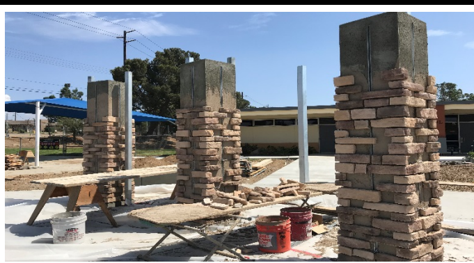
Stone veneer on columns
