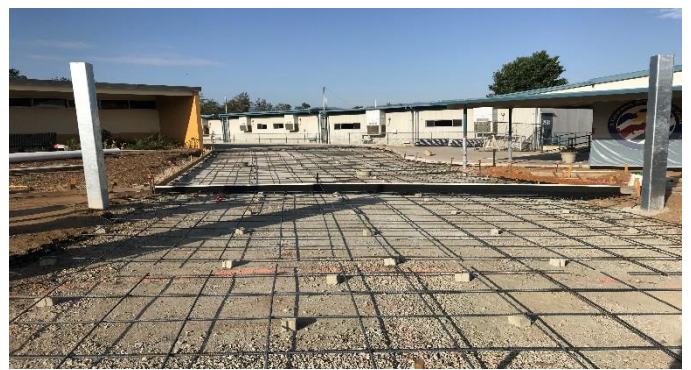
Rebar installation
