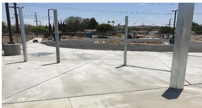
Concrete at fire lane & sidewalk
