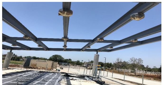
Lunch shelter paint prep
