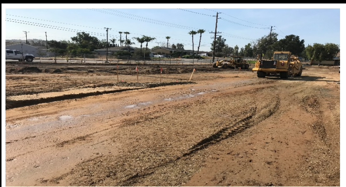
Front parking grading
