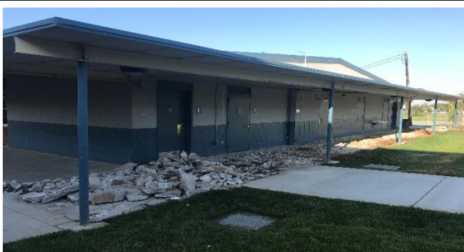
Building 2 concrete demo
