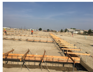
Area A-D Footing Form Work
