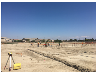
Area F-G Rebar and Form Work
