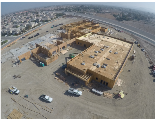
Area E Framing
