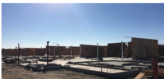
Area F-G Framing
